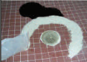
Floor Drains- use speedy dry, booms or drain covers to prevent oil from entering drains
