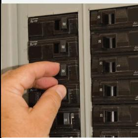
Locate the correct energy isolating device
